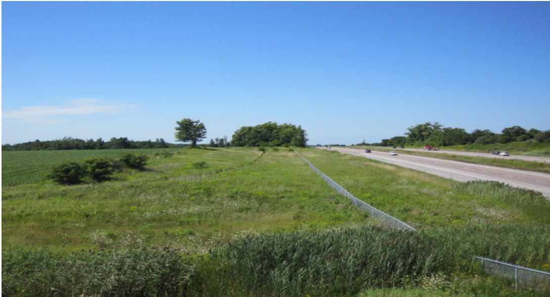
Photograph #24: Looking west from Sideroad 24 along the proposed transitway corridor route.
