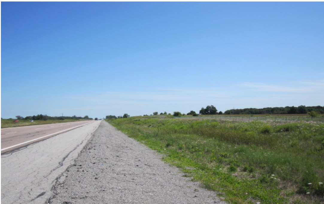
Photograph #21: Vacant lands associated with the proposed transitway corridor east of York Durham Line.
